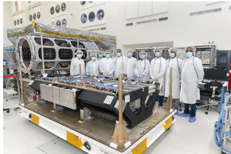
NISAR Team Preparing for Installation of the ISRO S-SAR Instrument on the Radar Instrument Structure (RIS)
